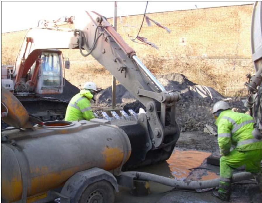
**Tar treatment:** Contractors excavate the tar tank at the Salford Gasworks before the tar-impacted fill is stabilised and solidified (above) using ScotAsh products. All pictures courtesy of Eneotech Environment Ltd
