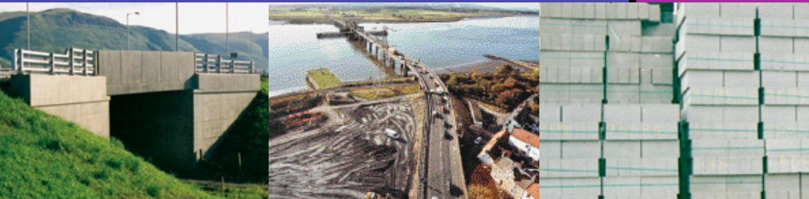
ScotAsh FBA has been used as backfill for bridge abutments in Clackmannanshire and Fife and in the manufacture of lightweight building blocks
