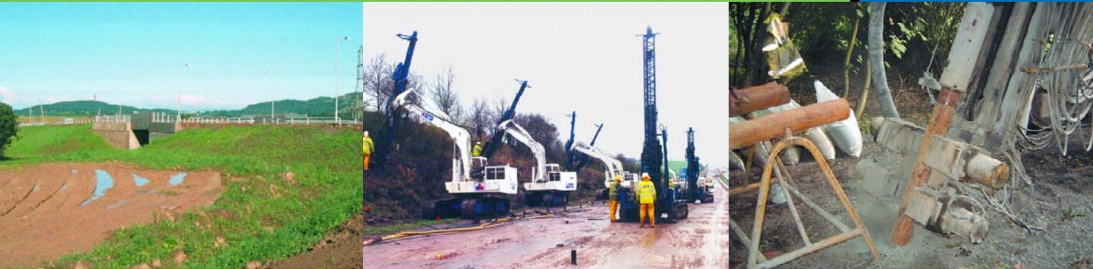
Conditioned PFA has been used as lightweight fill for the Tullibody Bypass, for grout manufacture for mine filling on the M8 and filling abandoned mines
