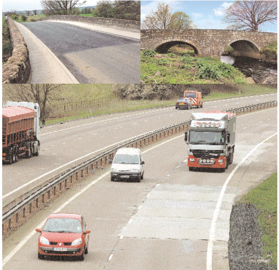
*Superpozz SV 80 was used to strengthen Eden Bridge (top photos) and to repair the M90 carriageway*
